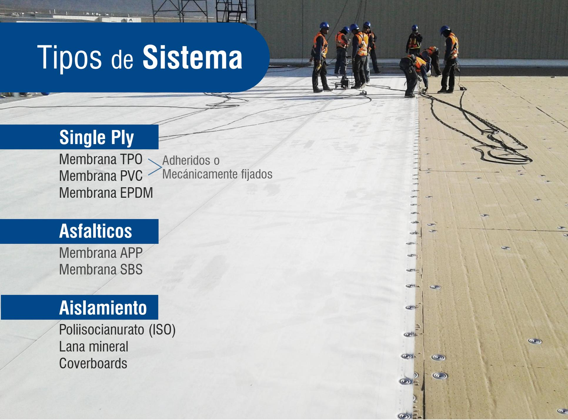
A wide-angle photograph of a construction site on a flat roof. Several workers in orange safety vests and blue hard hats are working on a large, light-colored membrane. The membrane is laid out in long, parallel strips, with some sections already secured with metal fasteners. The workers are positioned in the background, some standing and some kneeling, engaged in the installation process. The sky is clear and bright, suggesting a sunny day.
